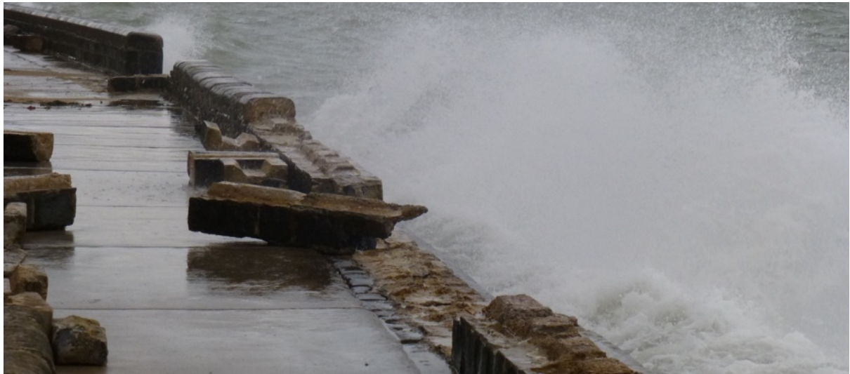
Figure 10. Destructive wave action: In June 2014, storms coinciding with high tides caused havoc along Bayside beaches. Large slabs of basalt, some weighing several tonnes were thrown for more than two metres by the waves. This site is along the sea wall between Blackrock and Ricketts' Point.
